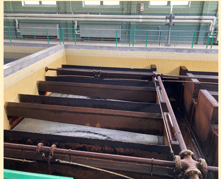
Filter Down for Maintenance
