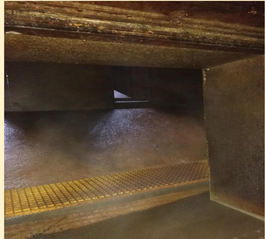
North Plate Settler Inlet
