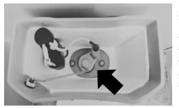
One of the most common culprits and leaks not always heard is the leaky toilet flapper in the tank, which can leak water 24/7 or intermittently (see the arrow on the image to the left). The flapper may seal okay on one flush, but not tightly on the next. We developed a short "how to" video demonstrating how to do a dye test on your toilets to find out if a flapper needs flipping. Find it on the Common Service Issues page.
