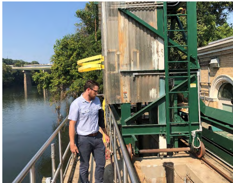
Figure 4. Troy Belcher inspecting the Queen Lane Raw Water Intake Coarse Screening Equipment as part of the intake upgrades and screening evaluation. HDR will use lessons learned from from intake facilities and operations for consideration on the Big Lehigh Intake.
