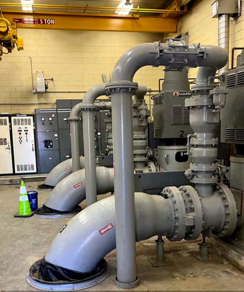
Figure 2. Existing PARCO Operated Valve and Air Release Valve on Pump #3 Discharge
