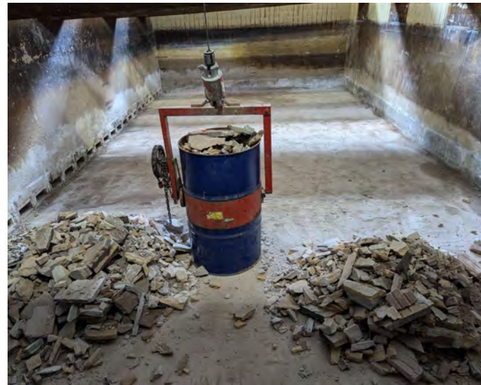
Filter #1 Media and Underdrain Demolished
