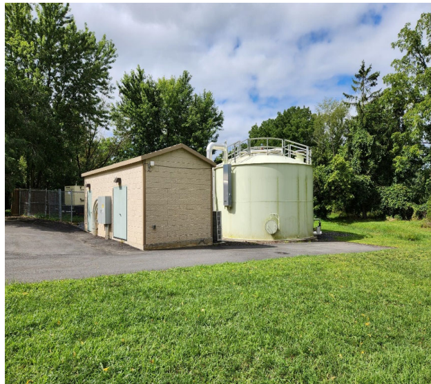
Control/Chemical Building & Tank
