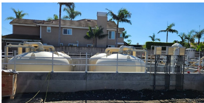
AECOM recently constructed a PFAS treatment facility in California that took this approach due to construction within a residential area so that the tall pressure vessels would not impede the surrounding viewshed.
