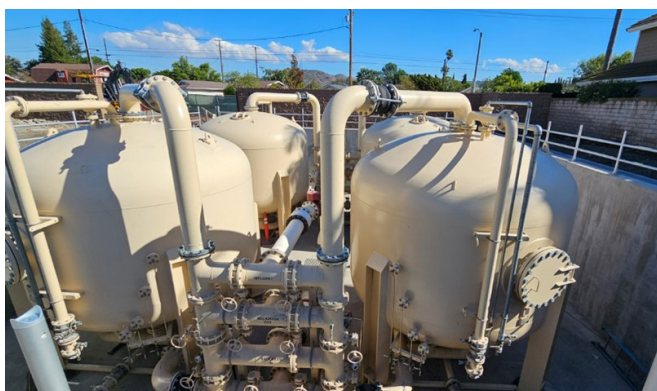
AECOM recently constructed a PFAS treatment facility in California that took this approach due to construction within a residential area so that the tall pressure vessels would not impede the surrounding viewshed.
