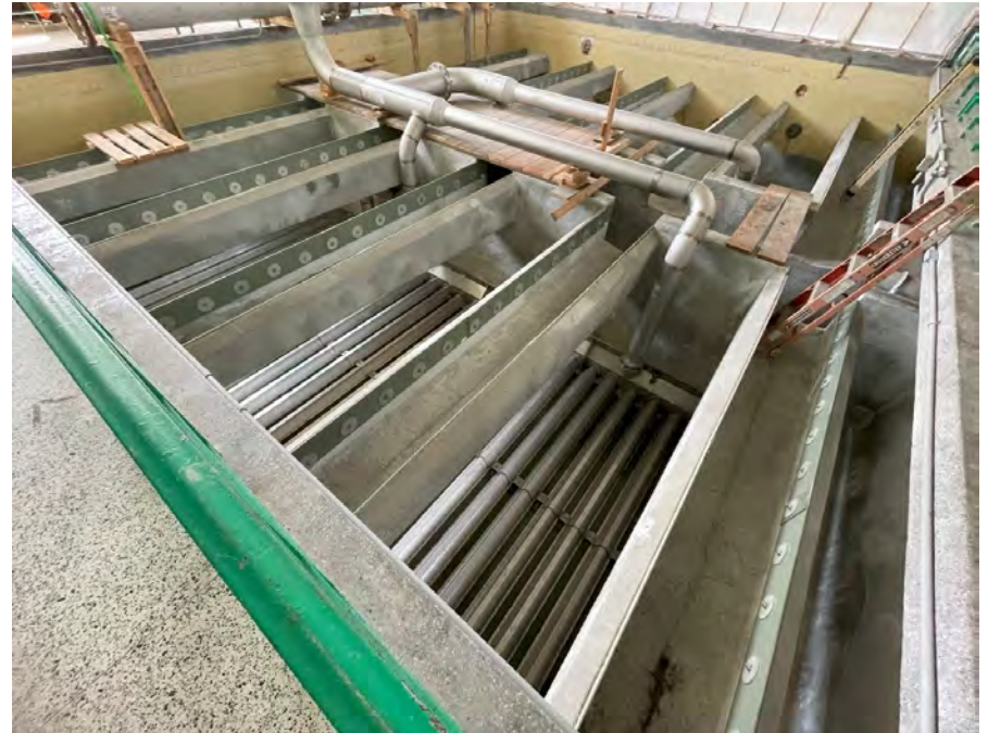
Filter #1 ready for media placement
