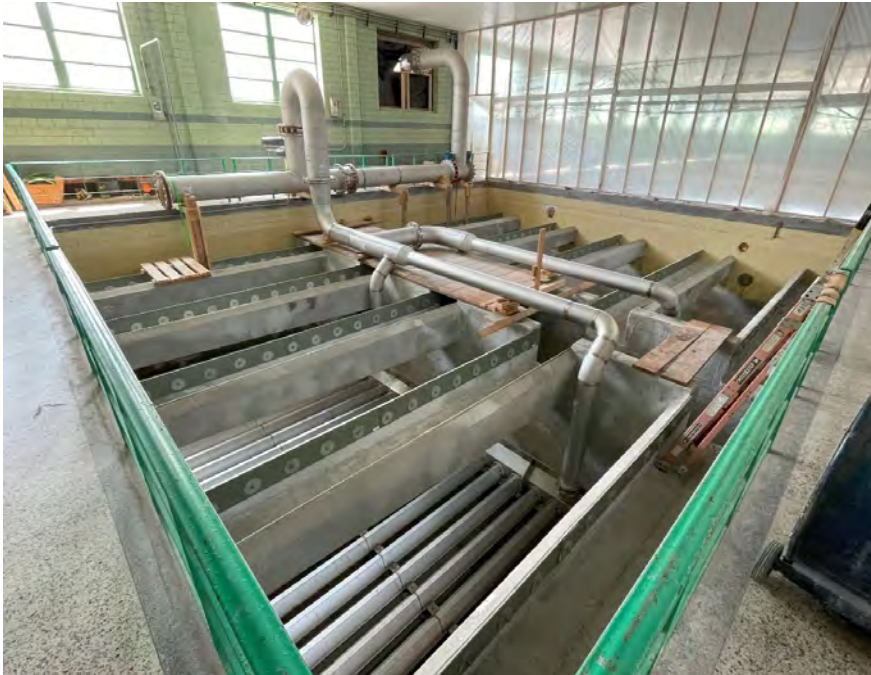
Filter #1 new underdrain
