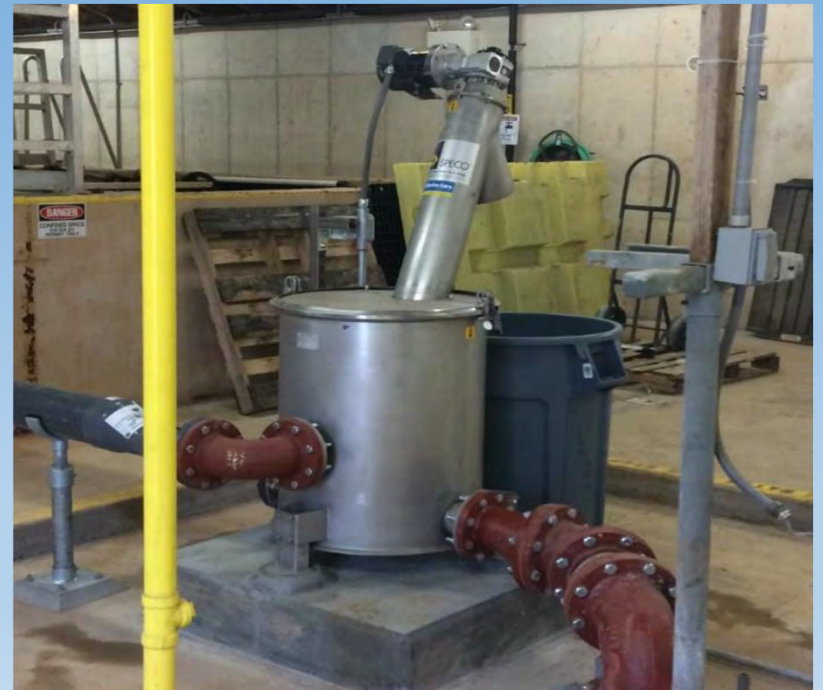
Compact screw type screen for pumped raw wastewater
