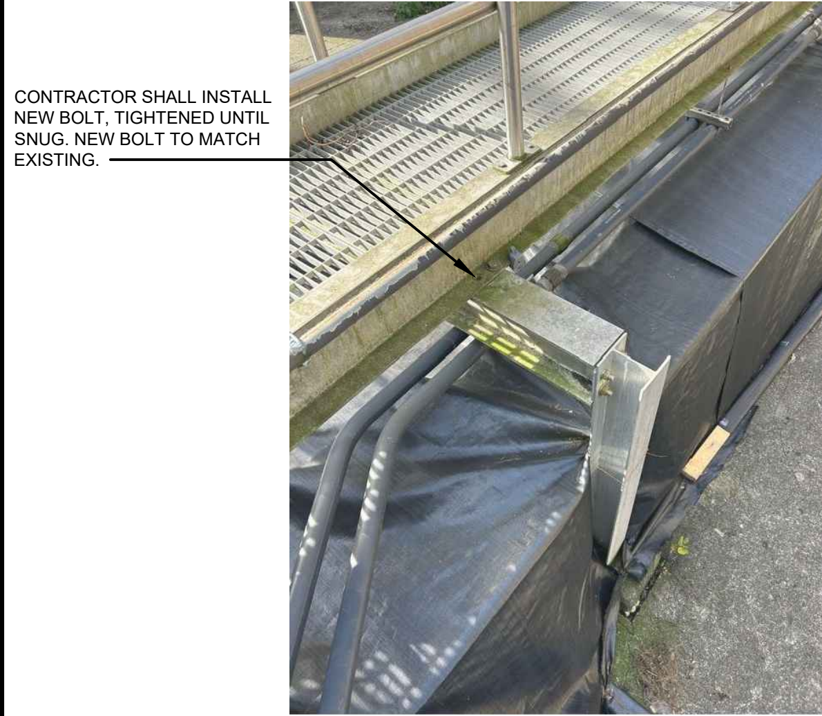
1 PHOTO OF MISSING BOLT SCALE: NONE
