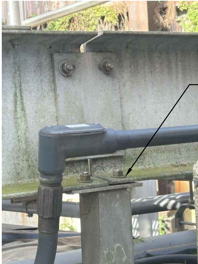
2 PHOTO OF LOOSE BOLT SCALE: NONE
